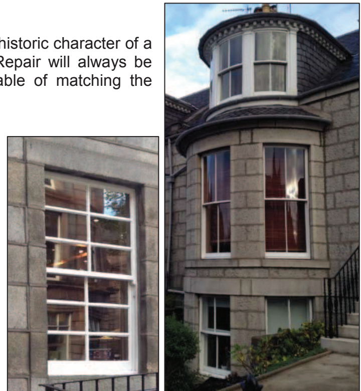
Examples of rectangular panes and curved glass
