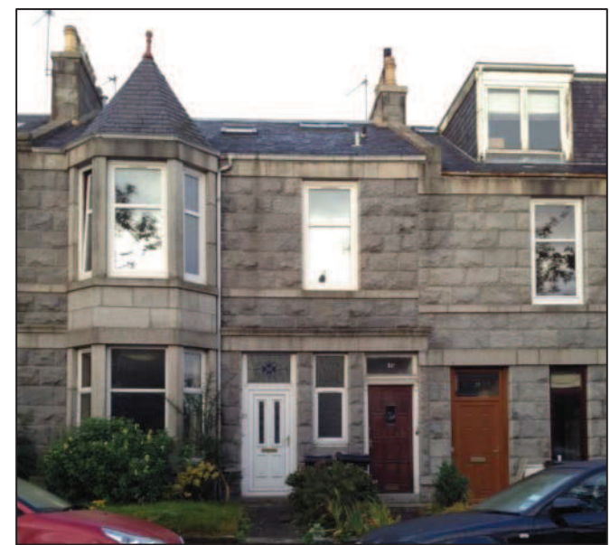
Inappropriate change can negatively affect streets and wider areas as well as individual buildings
