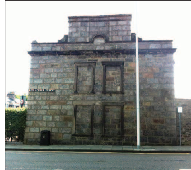
Example of blocked up windows in Ferryhill
